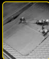
Battery protection with strap
